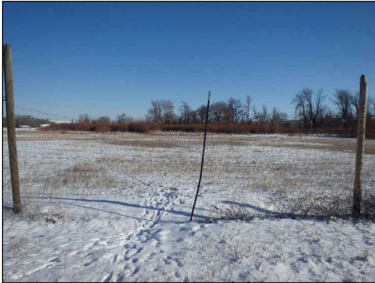
Damaged portion of Heart K fence
