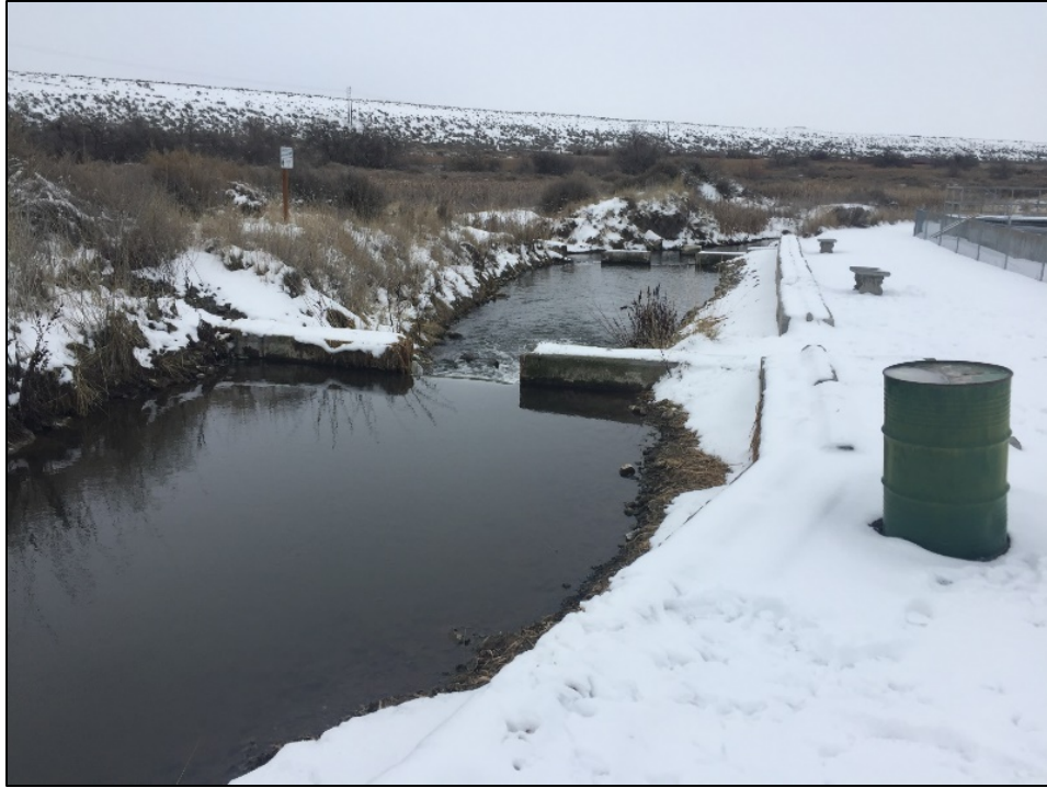
Fishing area at low water. Boards are installed to develop fishing ponds.
