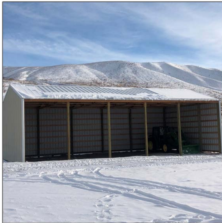
New equipment storage building completed at Scotch Creek headquarters - Photo by Jim Olson
