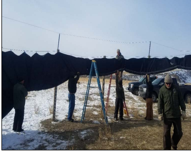
Feb. 7: WDFW staff members help put the finishing touches on the Chelan Butte sheep trap
