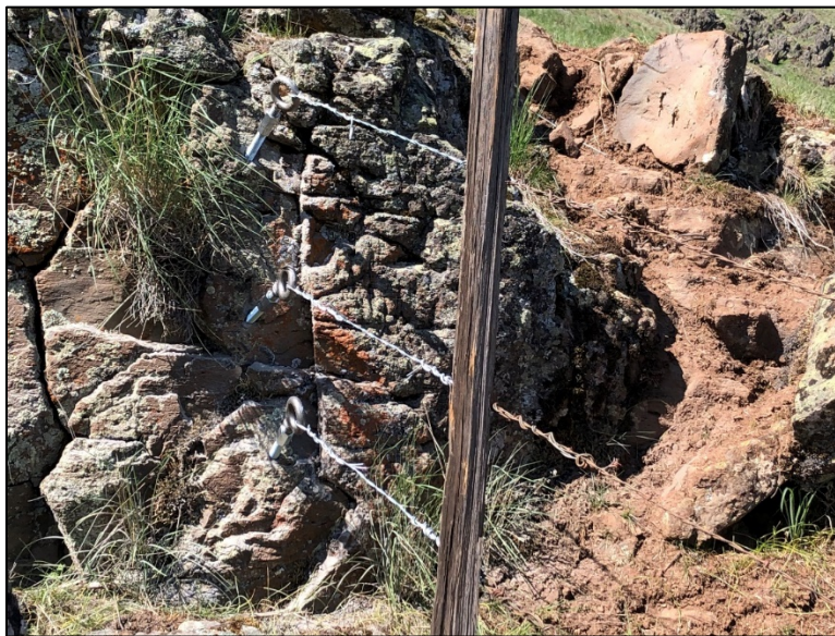
Installed eye bolts in the rock to anchor wire
