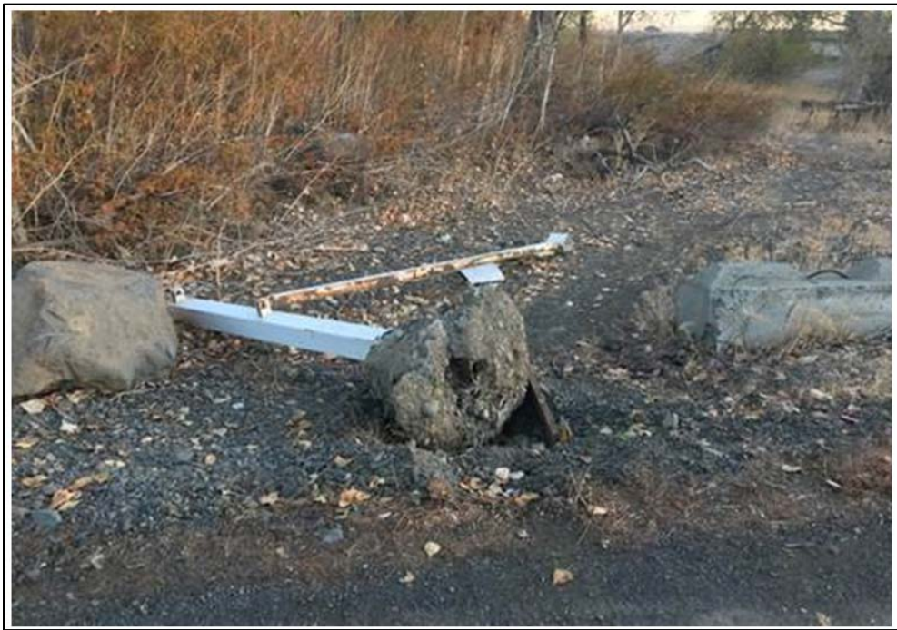
Vandalized gate at Zillah Bridge
