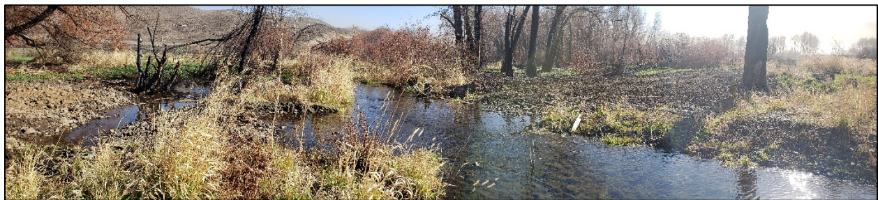
Mellotte bridge site after removal of bridge and fill material
