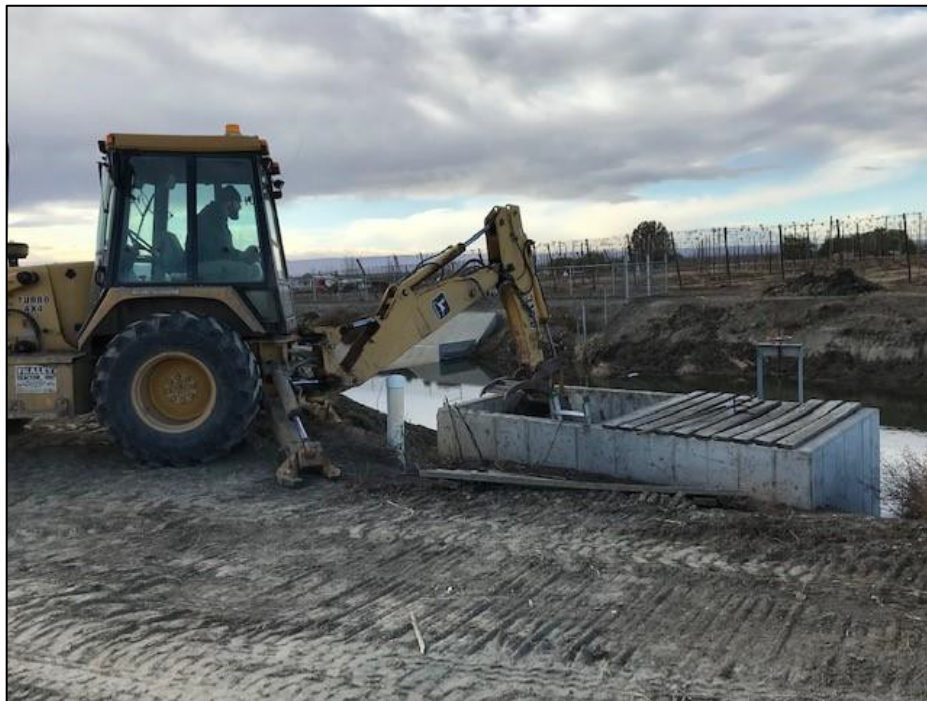
Lifting debris out of the Sulphur Creek diversion weir box
