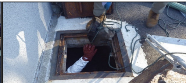
Martin access site boulder removal
