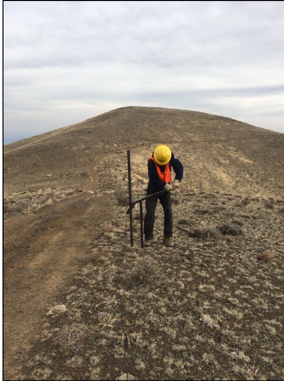
WCC worker pulling t-post
