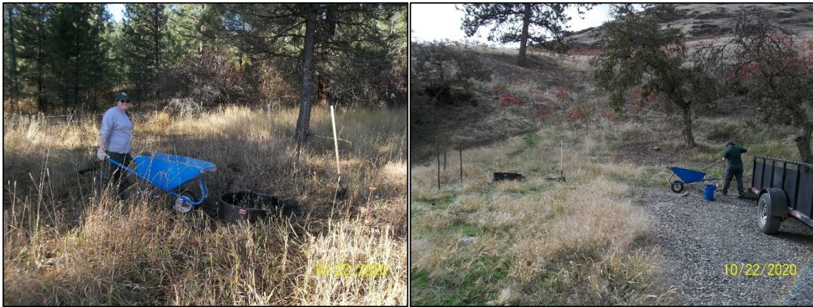
Heimgartner and Wight installed fire rings at campgrounds
