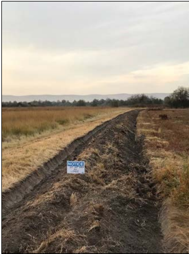
Signage to discourage walking on and trampling down new leve
