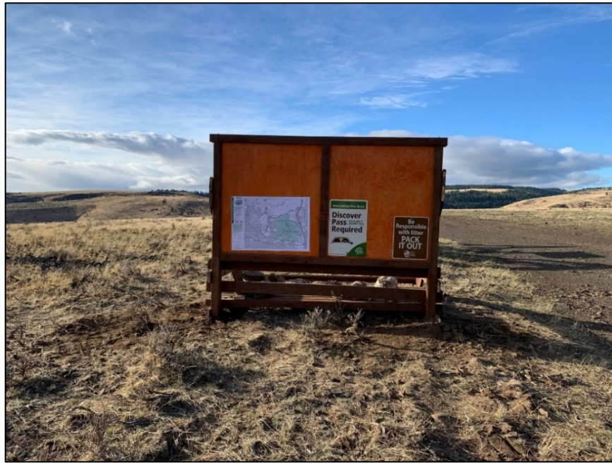
Erecting the Beacon Ridge kiosk built by Boy Scouts
