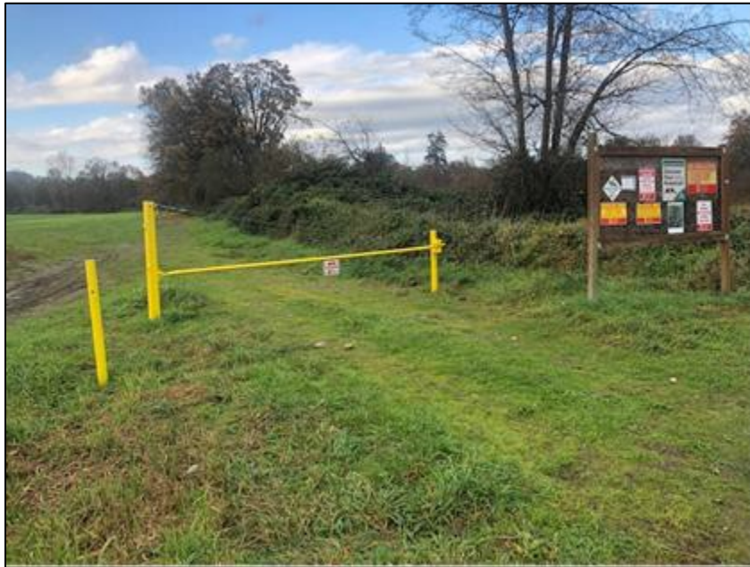
Example of repaired and painted access gates and unit entrances
