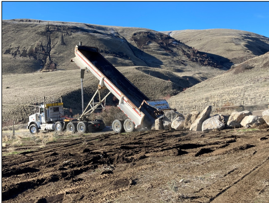
Barrier rock being delivered to Colockum Wildlife Area
