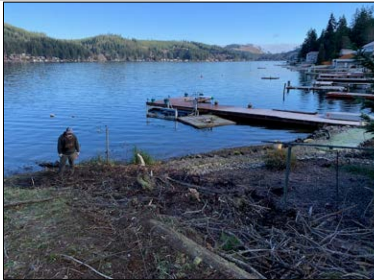
Summit Lake Trees and Damaged Fencing Removed
