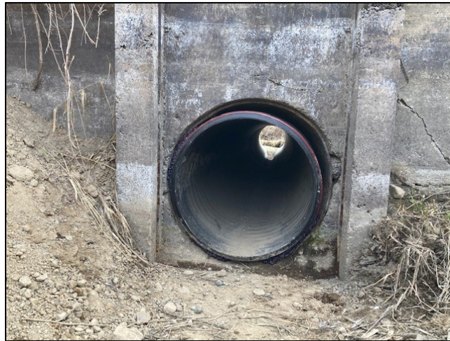
New culvert pipe seated in place
