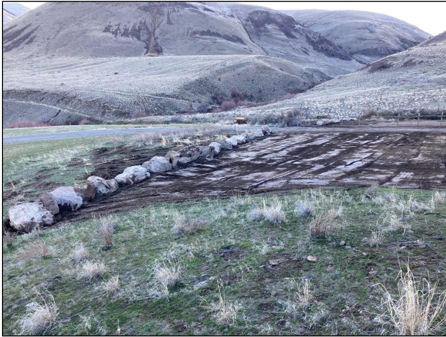
Barrier rock moved into place at Colockum Wildlife Area Headquarters
