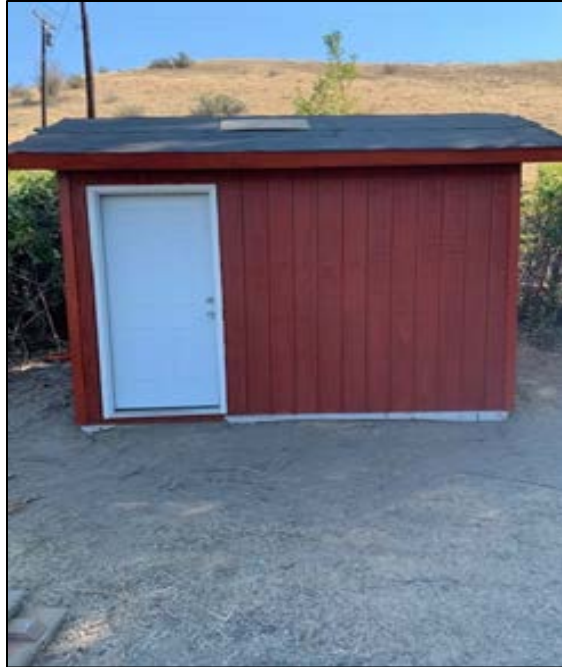
New pump house built by Wenas team
