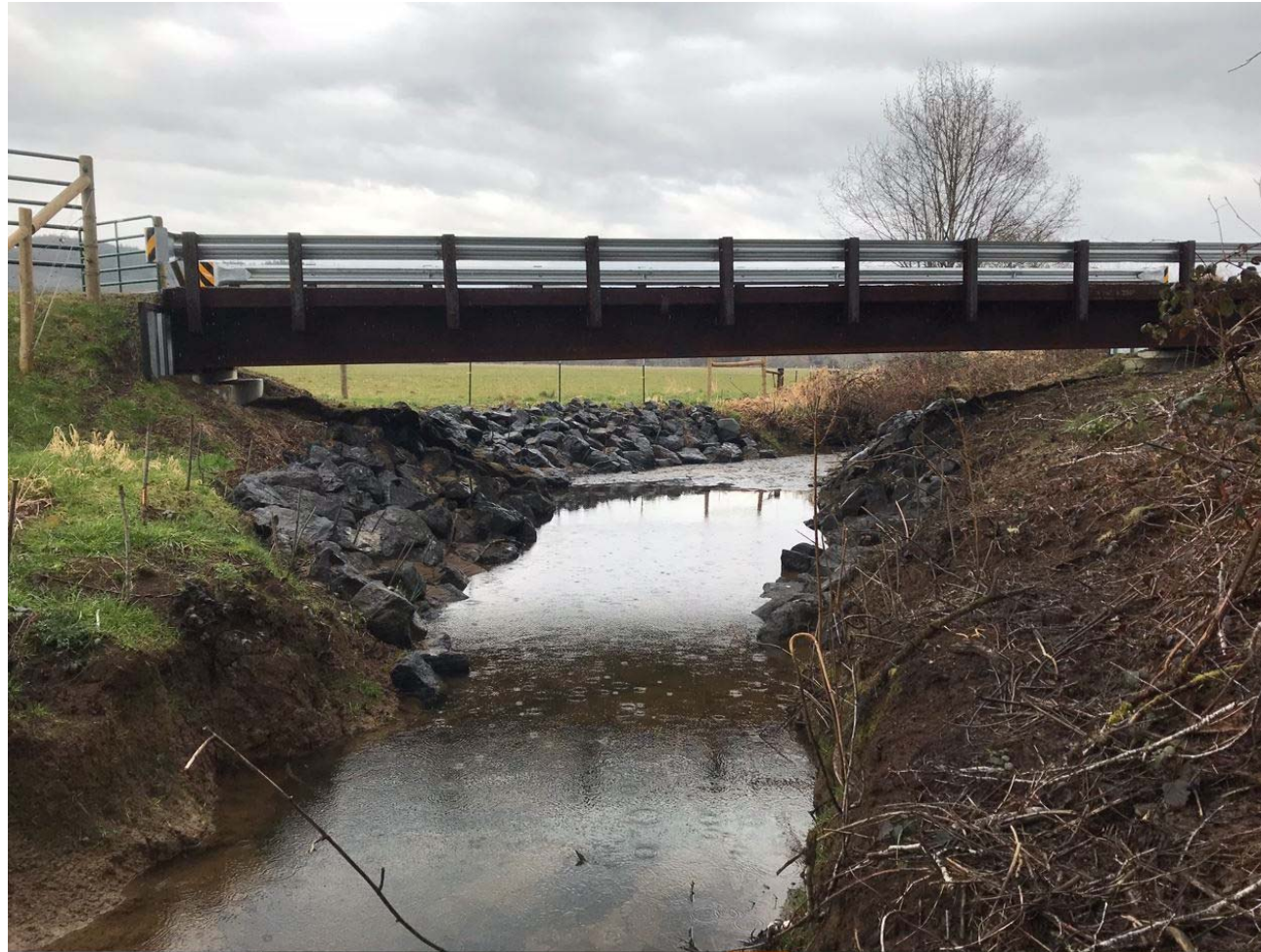
After: 60ft steel bridge
