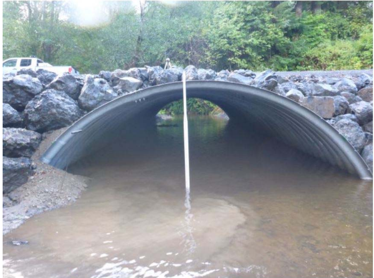
After: 19ft x 55ft arch culvert
