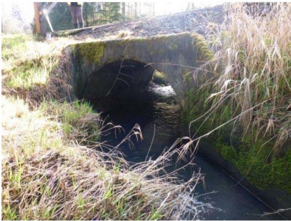
Before: 4ft x 45ft squash culvert
