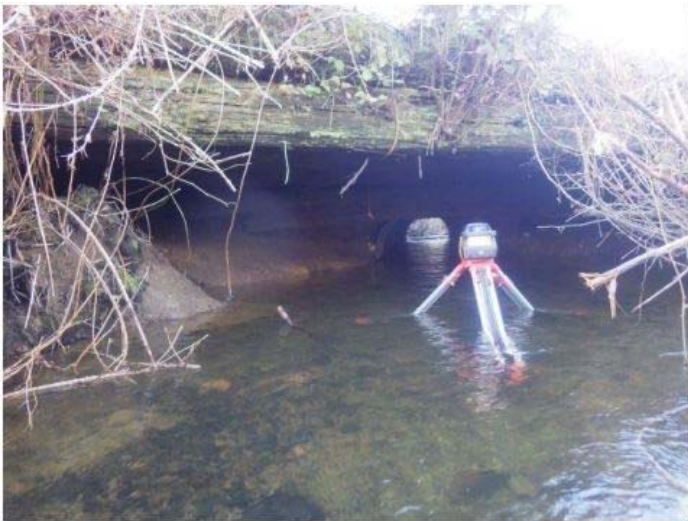
127Y0316 Before: 5ft x 40ft round culvert
