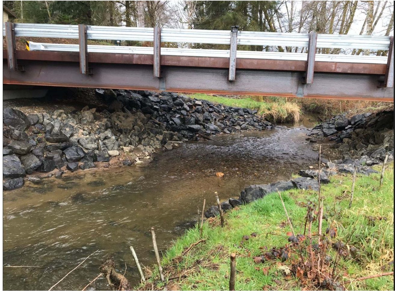
After: 50ft Steel Bridge
