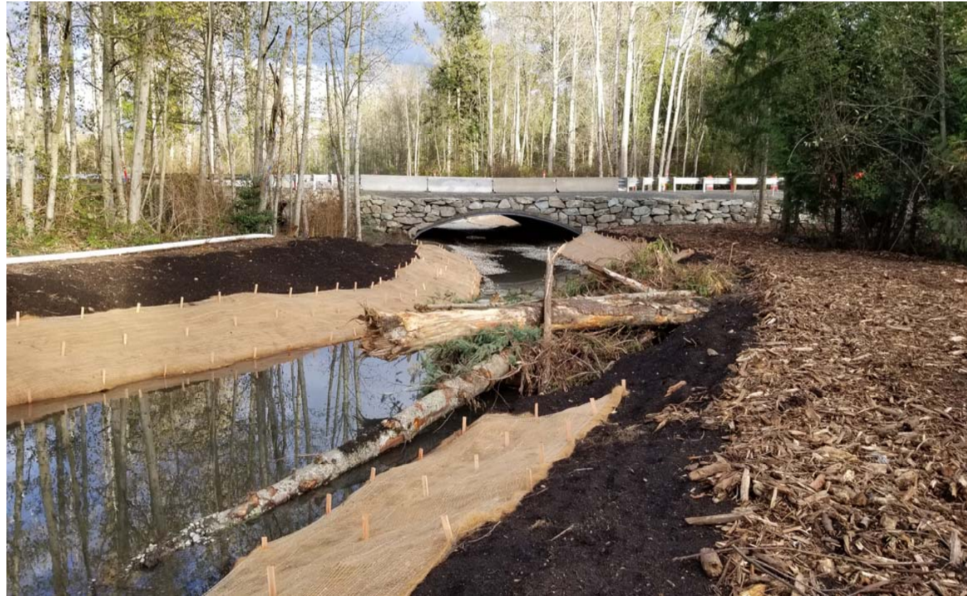
After: Bottomless Steel Plate Arch Culvert – 60 feet in length and 30 feet wide
