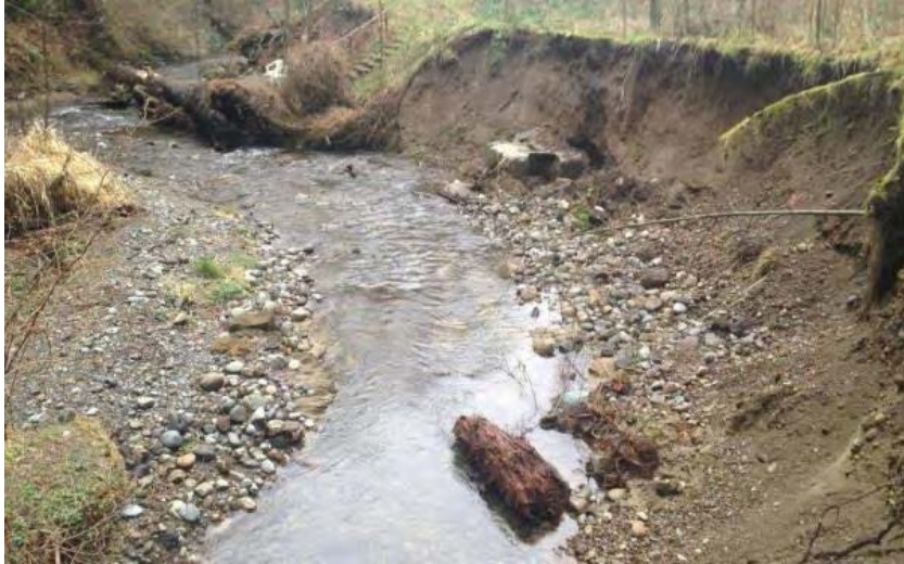
Photo of incised channel segment on Dickerson Creek downstream of failed log weirs (view downstream). Note box at toe of right bank is exposed septic basin. Photo by Tim Abbe, NSD (2/12/2013).
