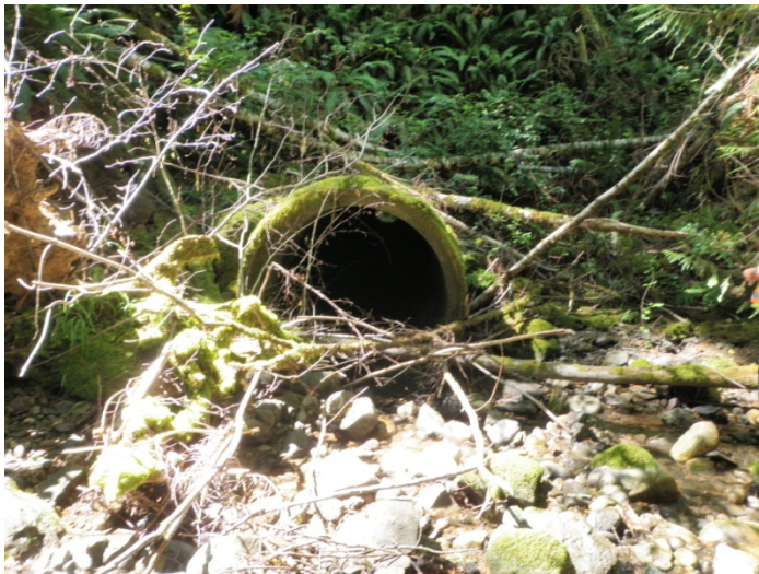
Photo at left shows a substandard culvert in the Hoko, below a restored area of the Hoko River.
