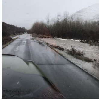
2-8-20 Watson Lake Footbridge
