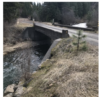
3-10-20 Cow Camp Bridge
