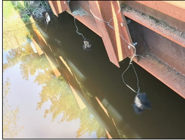
Strips of bear hide that will hang just above the water and hopefully deter the beavers from continuing to build their dam
