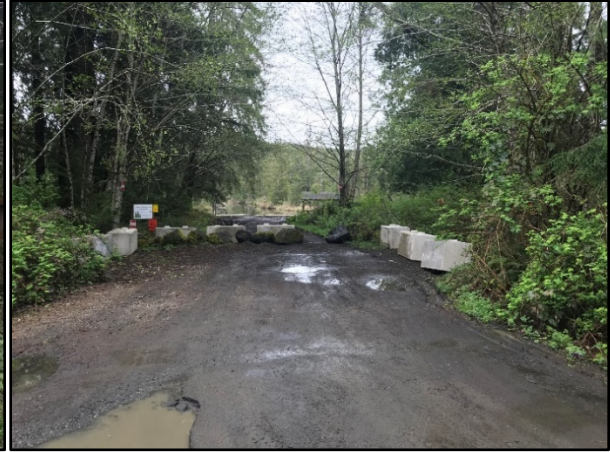
Ecology blocks in place to hinder further vandalism
