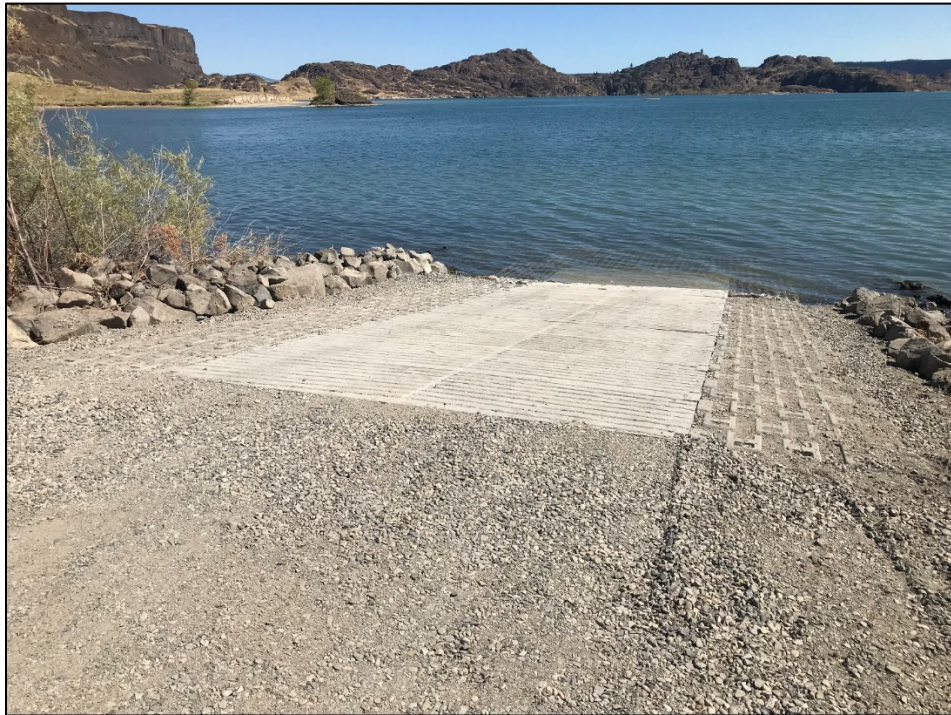
Barker Canyon ramp replacement
