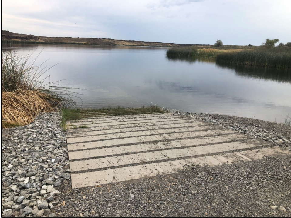
Burke Lake ramp repairs
