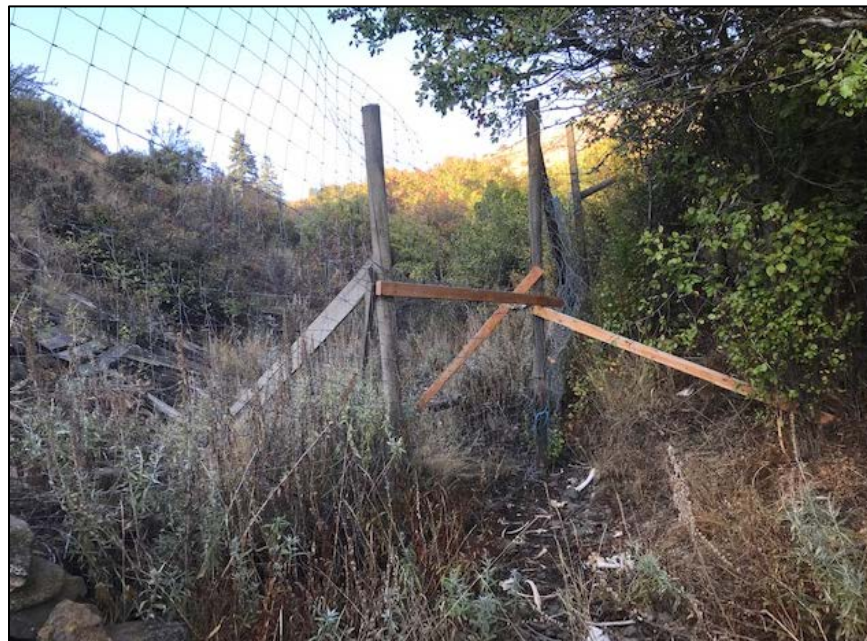
Coleman Canyon – a site that commonly needs some repair
