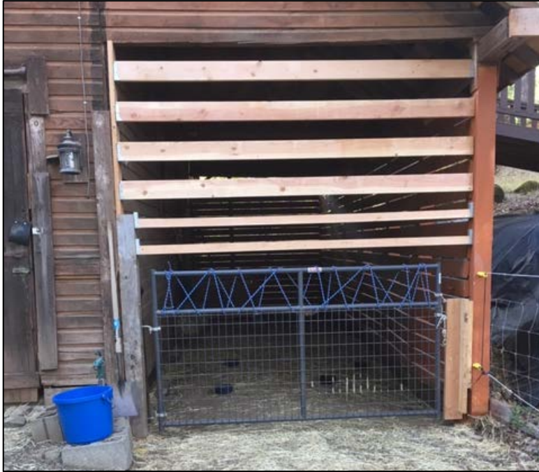
Goat pen under construction
