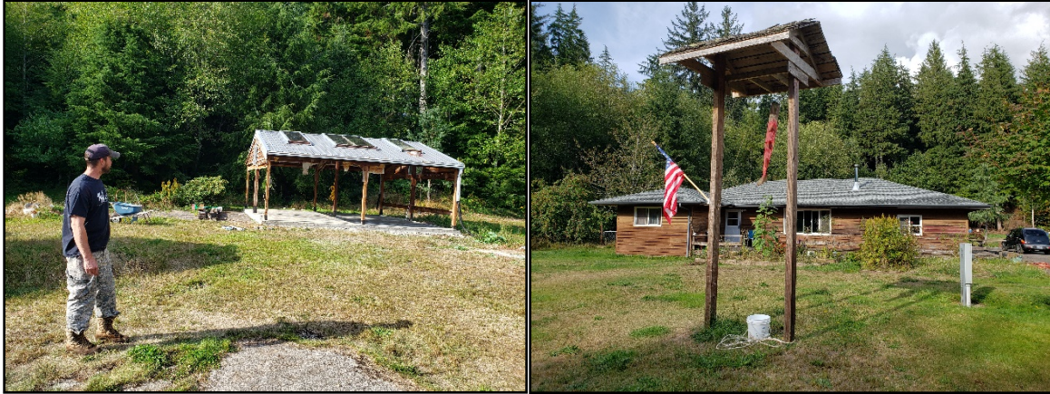
Structures on Sean Neuhauser's property near Forks which contain roosting bats
