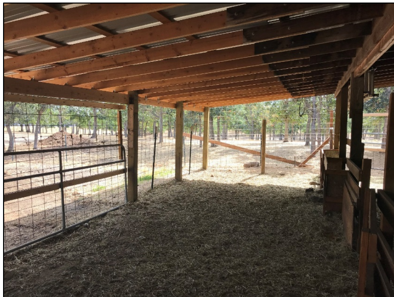
Sheep enclosure inspection
