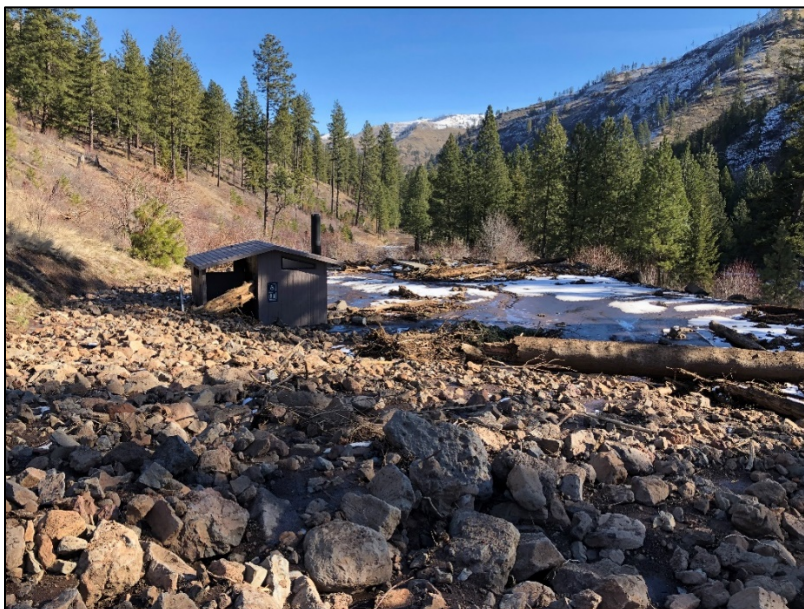
Destruction at Campground 9
