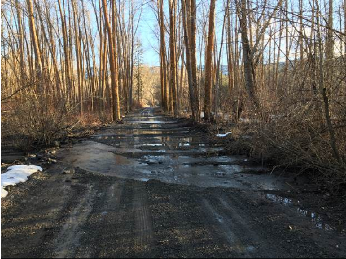
Water going over the roadway at Teanaway Junction
