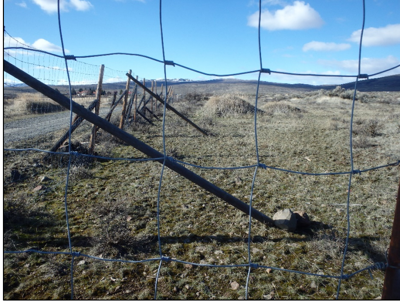
Section of the repaired fence near Cowiche
