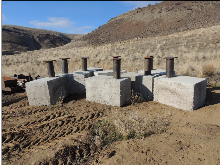
Large concrete footings used for gates
