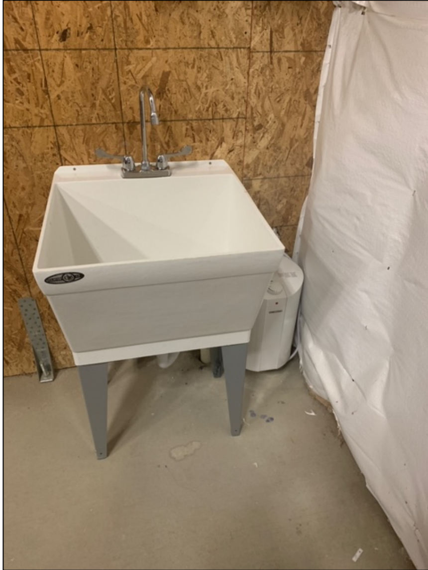
Water inside the shop!
