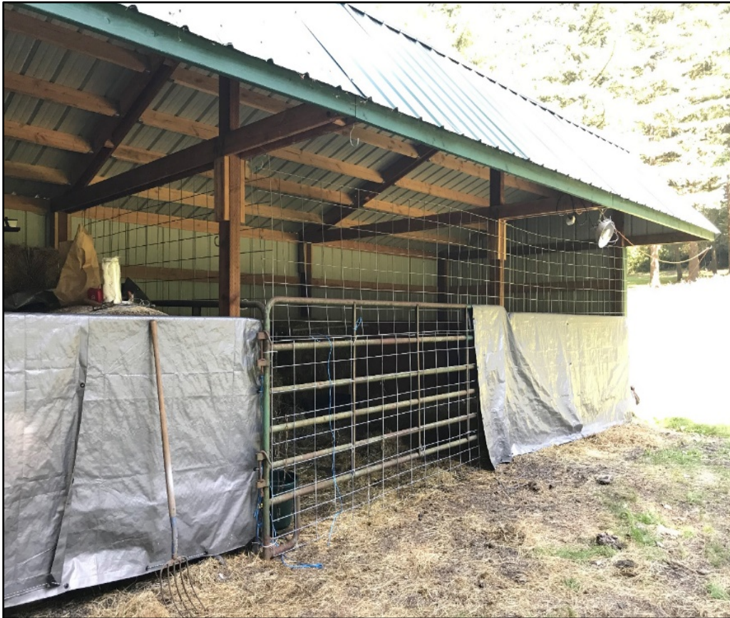
Landowner's night pen for the calf with hog-panel reinforcement installation in-progress
