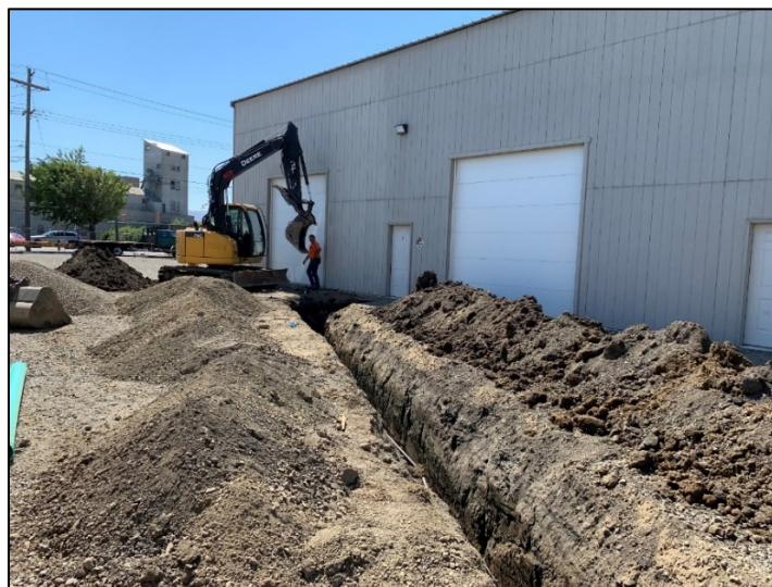
Ditch for water and drainpipe at WLA shop
