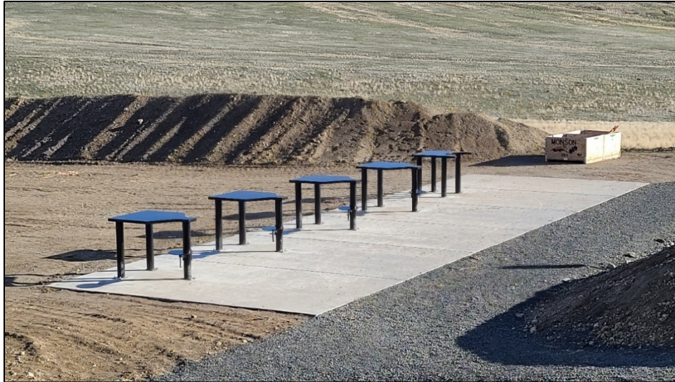
Some of the new benches installed at Sheep Company shooting range
