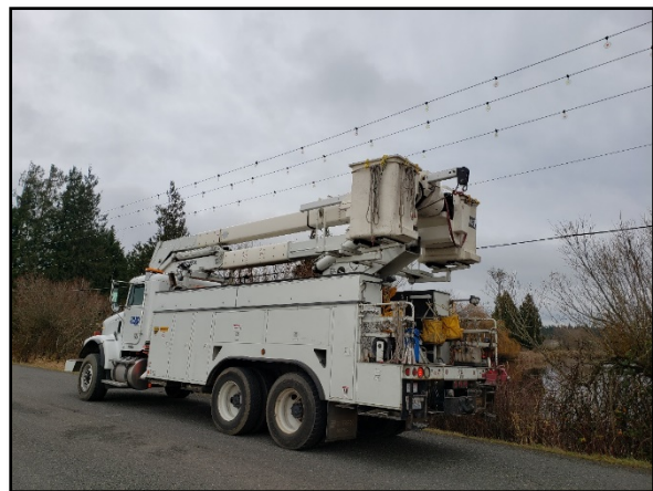
Fifty more diverters were installed but a line strike by a swan occurred the next day
