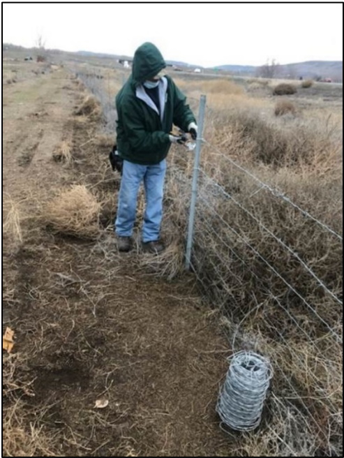
Natural Resource Worker Ruiz repairing fence along Pond 3 trail
