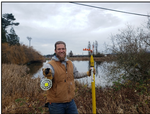
Clallam County PUD linemen respond to add more diverters to the lines
