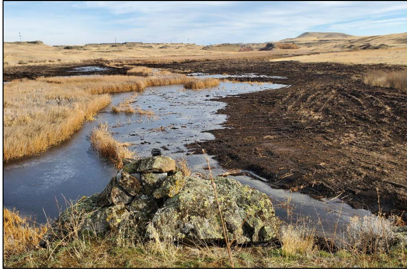
Revere Wetland Restoration Project (2020 image) post-restoration work with heavy equipment
