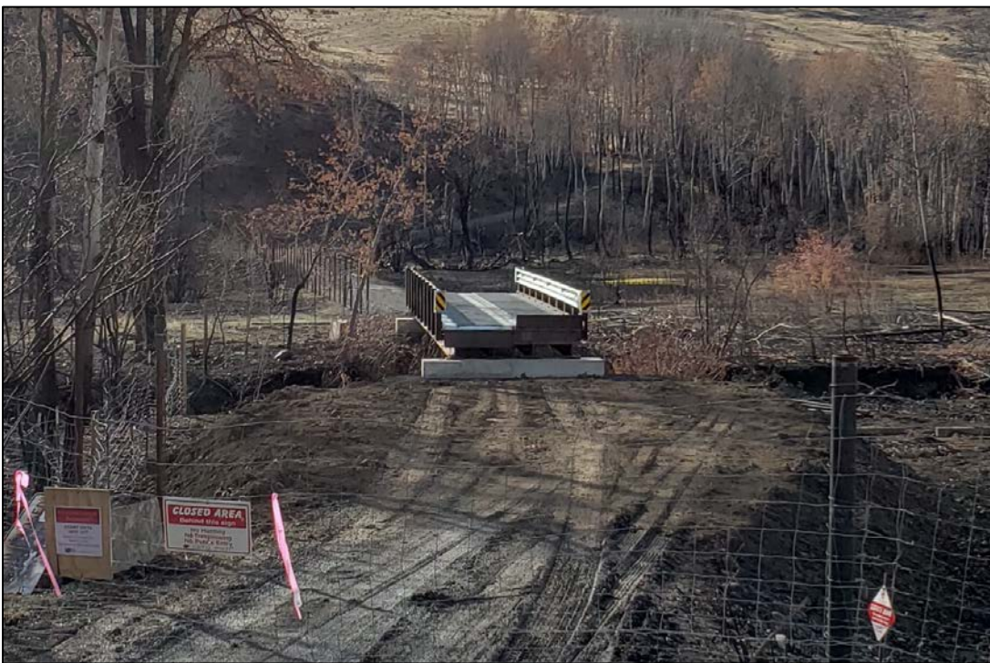
New bridge in place
