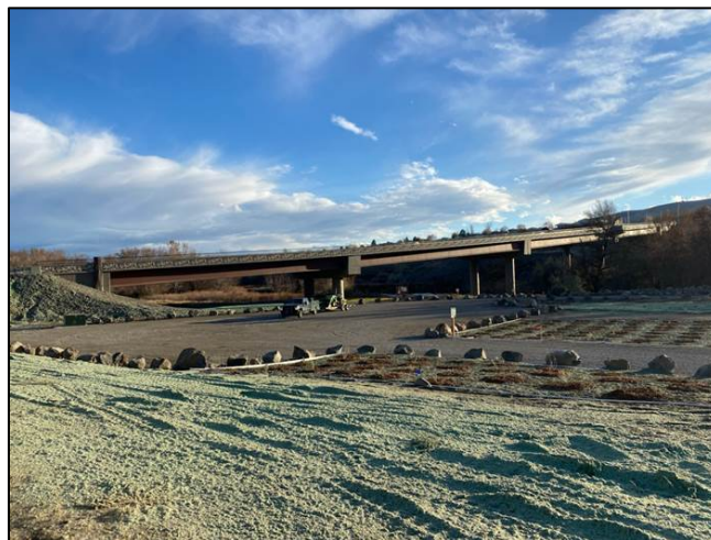
Duportail Access Site - New parking area
