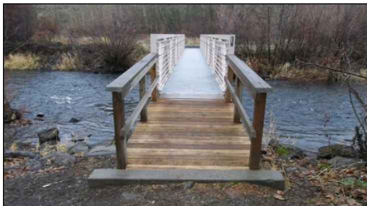
Replaced deck on the Watson bridge approach
