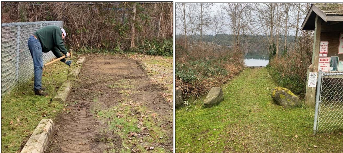
Barrier rocks installed
