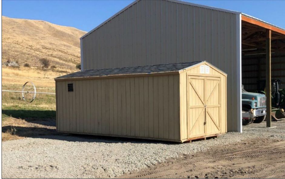
Scotch Creek storage shed moved to its new location — Photo by B. Dupont
