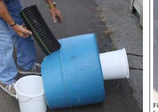
Figure 21. Insert the 6 x 16 in. drain line collar section 2-3 rings into barrel; affix firmly with adhesive, inside and outside of barrel. This needs to be solid.
