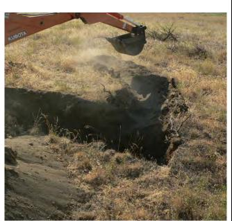
Trench for the burrow tunnel is done with a sweeping motion of the backhoe bucket. In this image it is a leftswinging and upward motion. This gives the trench an appropriate arc for the main tunnel. Some hand digging may be necessary (to get the trench deep enough) right where the main tunnel meets the collar/burrow chamber.
