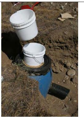
Figure 26. Finished burrow chamber, top buckets, and collar. Unit is being installed.
