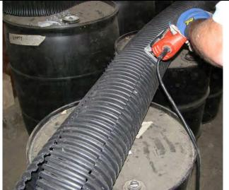
Figure 20. Cutting a 3-in. "walkway" in the 15 cm flex pipe with jigsaw (note: a jigsaw works best for this task).
