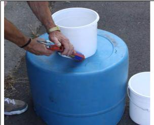
Figure 17. Use caulking gun to apply ample Liquid Nails (or similar adhesive) to solidly affix pail to barrel.
