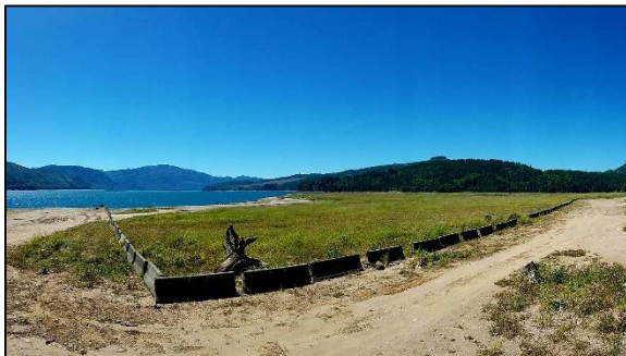
Figure 4: An ecology block barrier used to protect resources.
