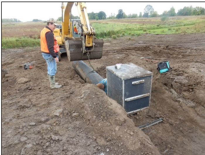
Figure 1: Installation of a new water control structure in the North Basin.
