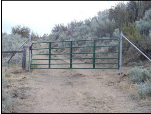
Figure 4: Gate with new pipe anchor points on either side.
