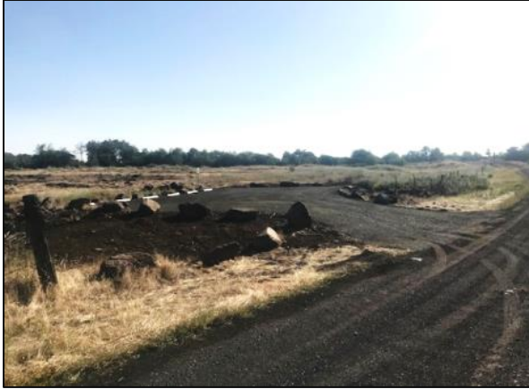
Figure 4: New, completed parking lot.
