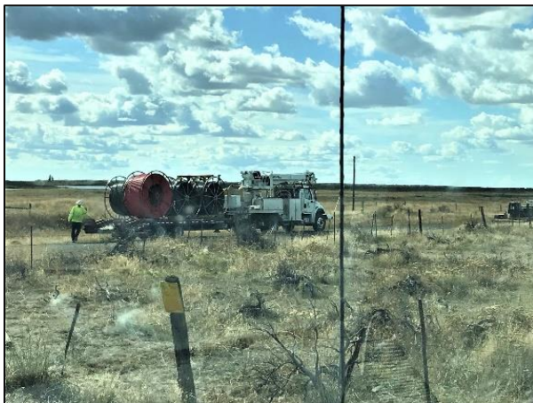
Figure 3: Crew burying power lines on the wildlife area.
