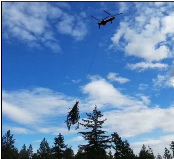
Figure 1: Helicopter flying in large woody debris
