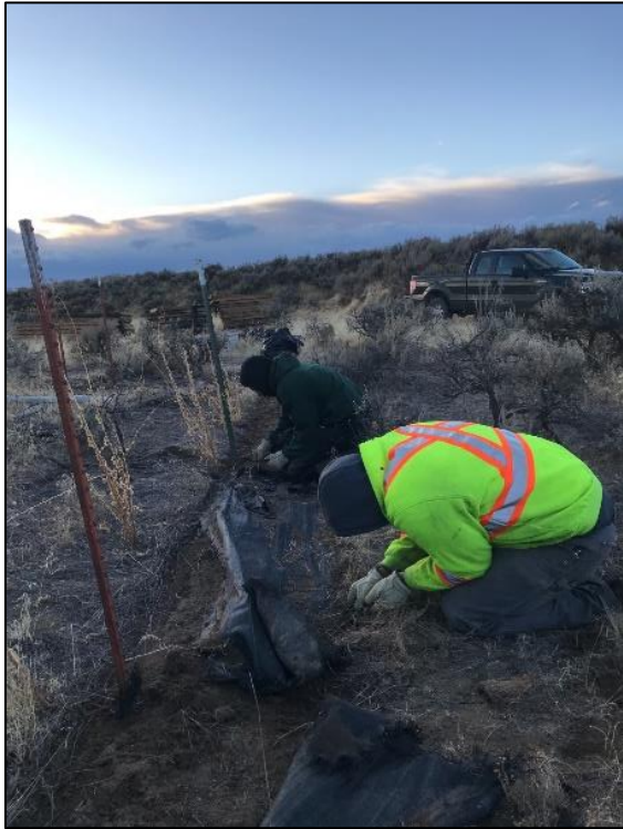
Figure 4: Pulling staples and fabric at the Tiny Town teardown
