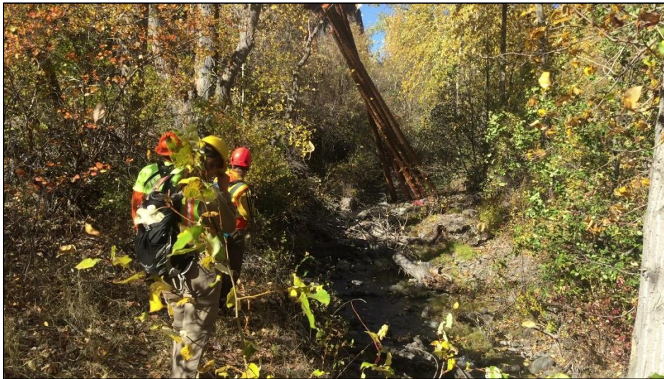
Figure 8: Crews placing large wood in Umtanum Creek
