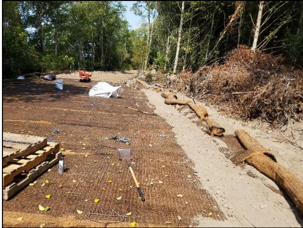
Figure 4: Nooksack Unit dike repair work
