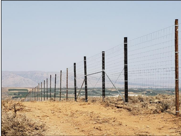
Figure 4: New fence built on the Cowiche Unit
