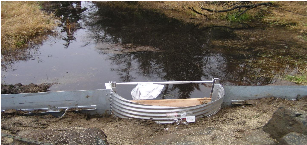
New water control structure on the John's River Wildlife Area
