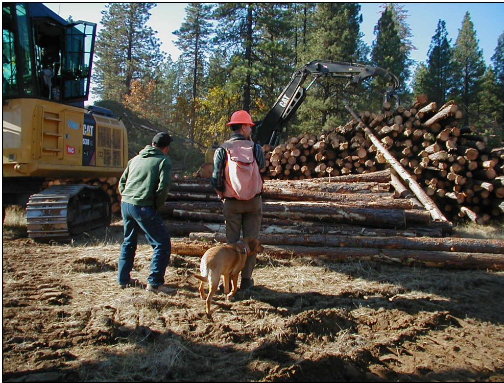
Observing forest thinning on the Soda Springs Unit
