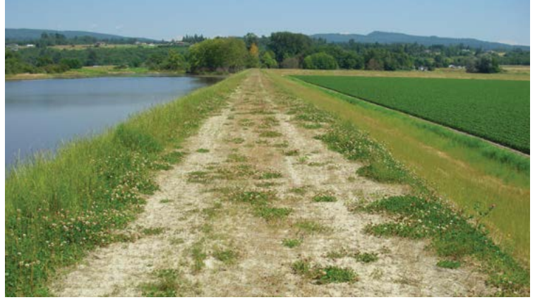
A levee protects adjacent farmland from flooding.
