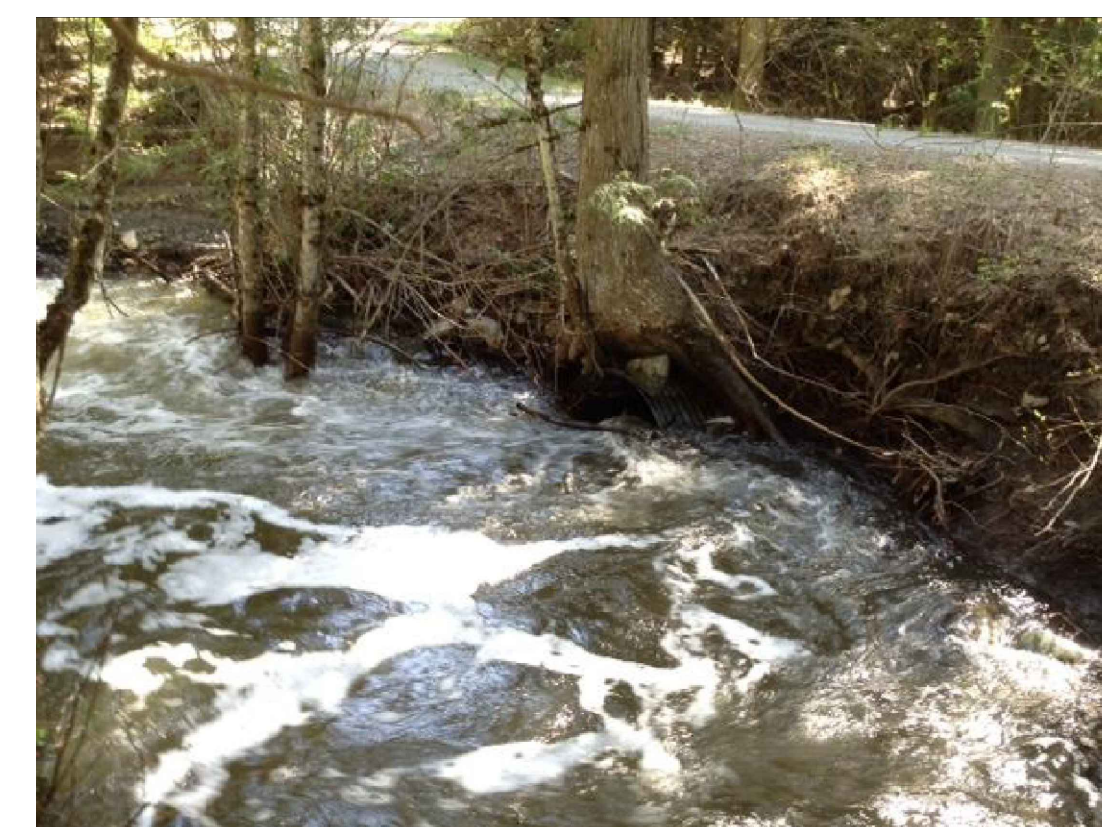
Inlet (4/15/2016); tree is growing around inlet, 50% plugged with debris
