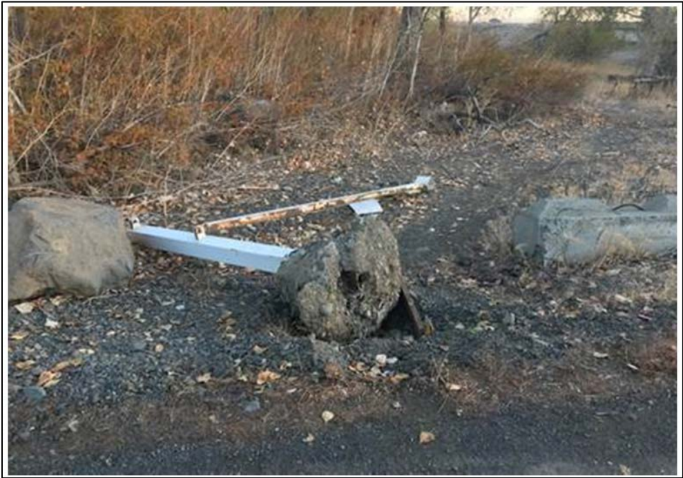
Vandalized gate at Zillah Bridge
