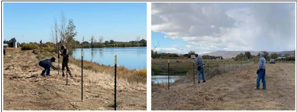
Access personnel replacing boundary fence at Pond 1
