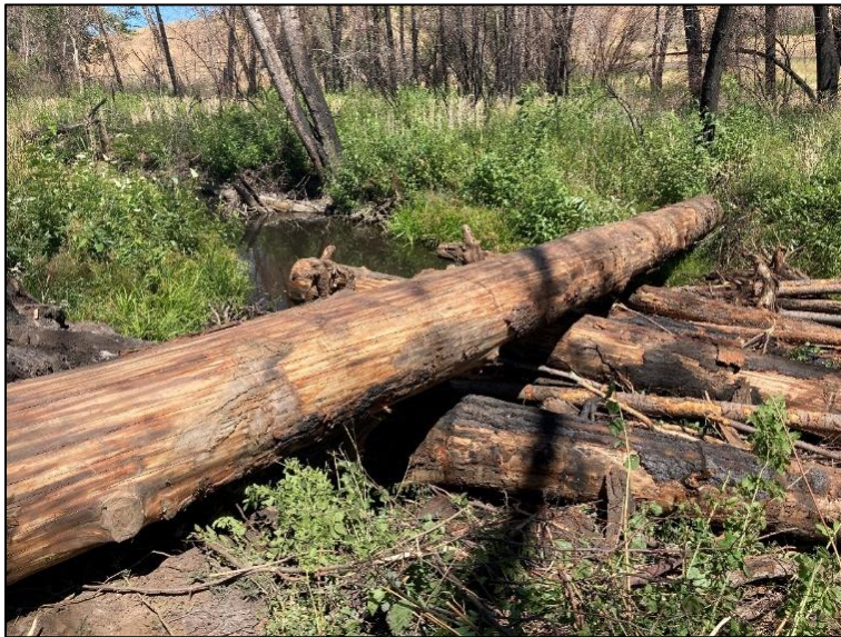
Log structures placed in Wenas Creek
