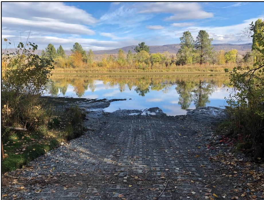
...and after construction
