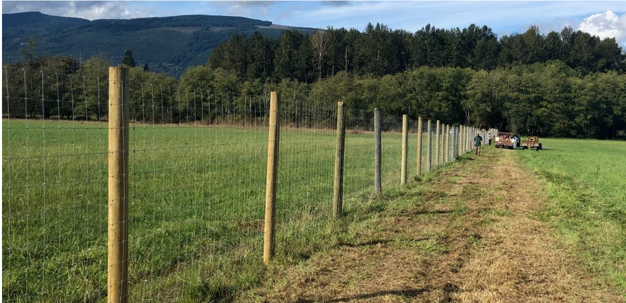
Figure 3. Fencing project in Day Creek
