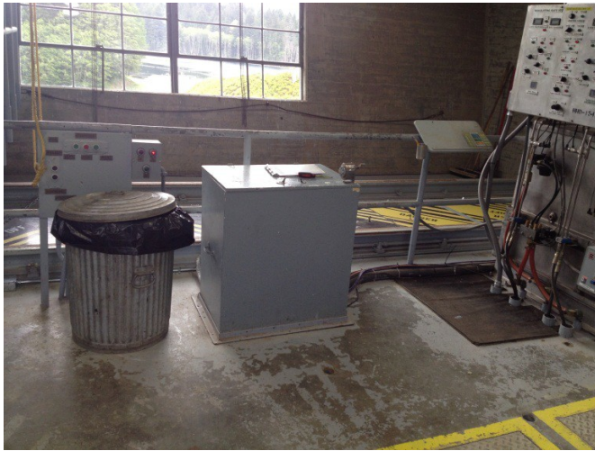
Figure 2. Outlet works intake tower reservoir level stilling well.
