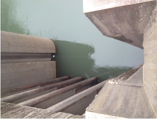
Figure 3. Mud Mountain intake upper trashrack structure.
