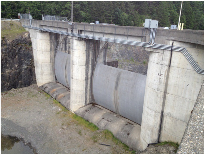
Figure 1. Spillway tainter gates at Howard Hanson Dam
