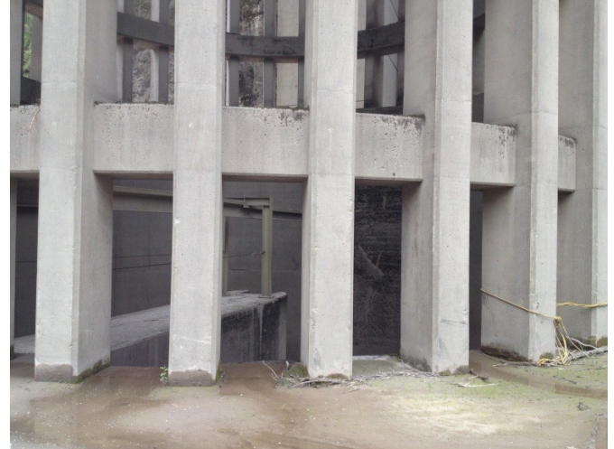
Figure 4. Lower intake structure stoplog slots.
