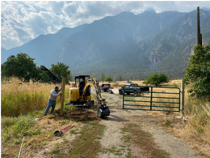
Staff installing a gate on the Chopaka Unit.
