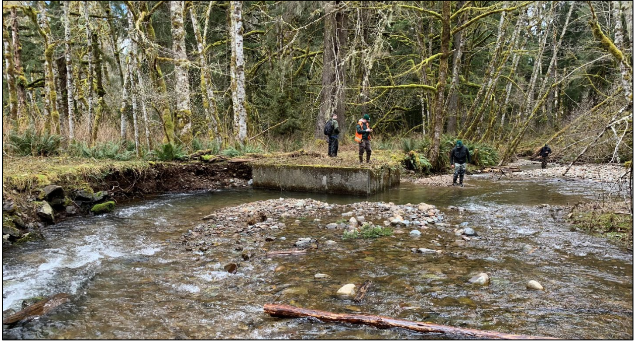
Alder Creek Diversion Structure.
