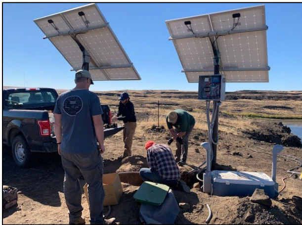
Staff replacing the Z-Lake aeration system, Sept. 2021.
