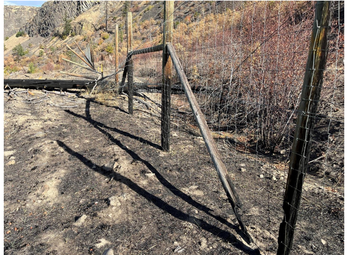
Elk fence damaged by Retreat Fire – Tieton River drainage
