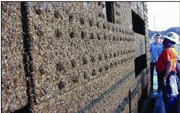
Invasive mussels fouling a penstock gate at Davis Dam. Photo by U.S. Bureau of Reclamation.
