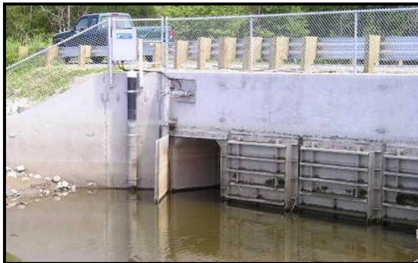
Figure 4-2. McElroy Slough Automatic Regulating Tidegate, “Aberdeen” style gate, open at a -2.7 foot tide event (County owned tidegate complex).
