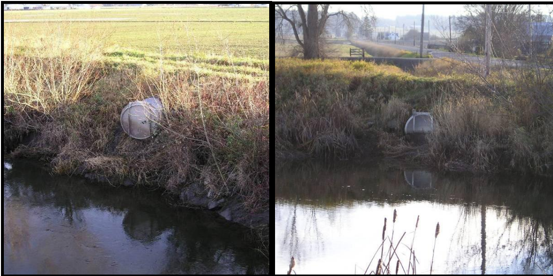
Figures 1-2 & 1-3 Floodgates, Drainage District 25 – Samish River system.
