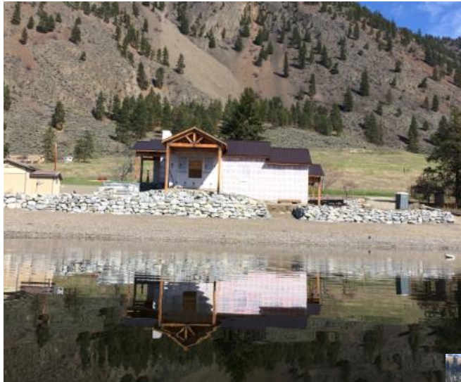
Violation 1 Unpermitted work to construct a newly hardened bank
