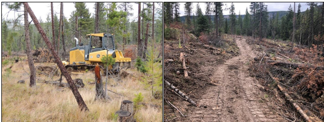
Fire lines being installed in preparation for treatment by prescribed fire
