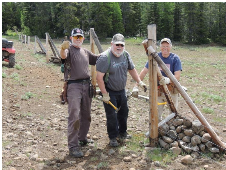
Rocky Mountain Elk Foundation volunteers repairing fence.
