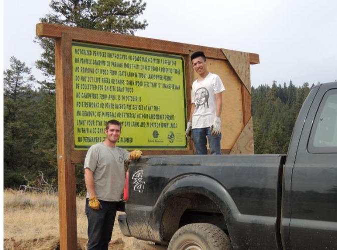
Colockum staff install a new green dot readerboard.
