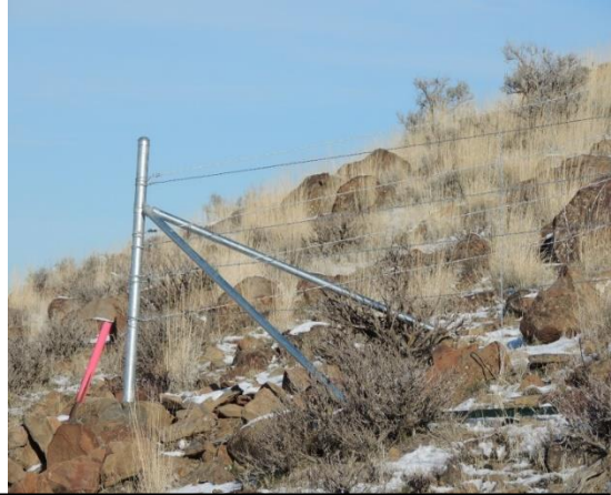
Fire-damaged fence corner, and a newly rebuilt, all-steel fence corner.
