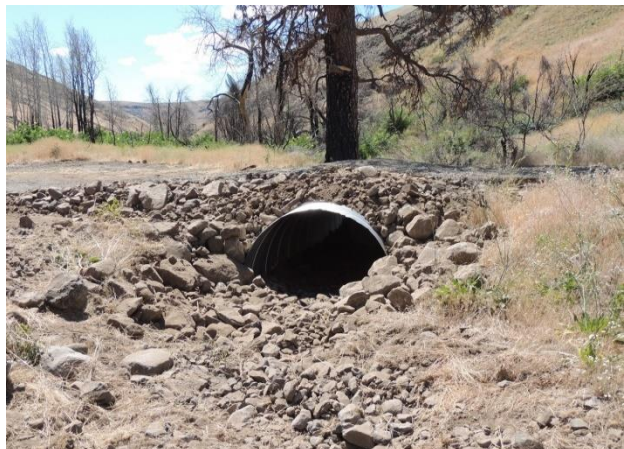
Drainage improvements on the Tekison Creek Road. Large culvert installed on Brewton Road.
