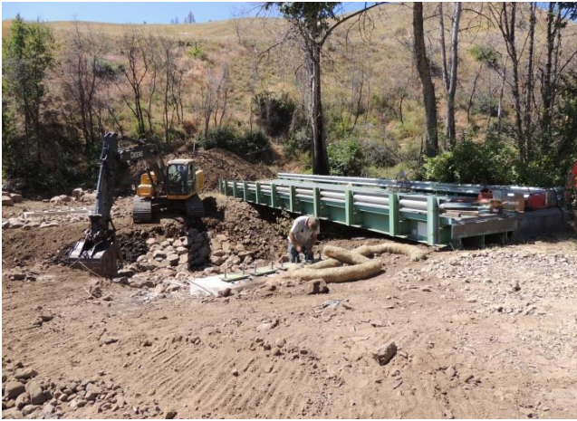
New bridge installation on the N. Fk. Tarpiscan Creek. Water drainage issues on the N.F. Tarpiscan Road.
