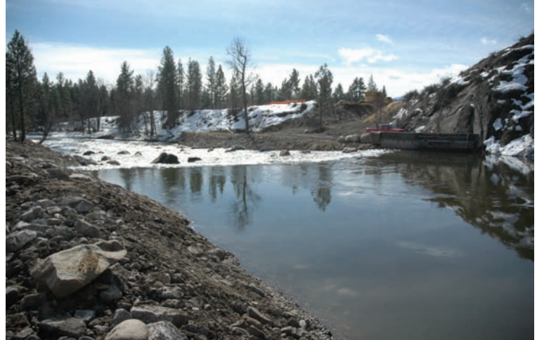
Fulton - completed structure looking downstream
