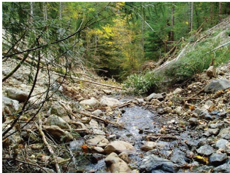
Brown Creek Decommissioning - Restored perennial stream channel following removal of road fill, culvert and placement of in-stream channel rock steps
