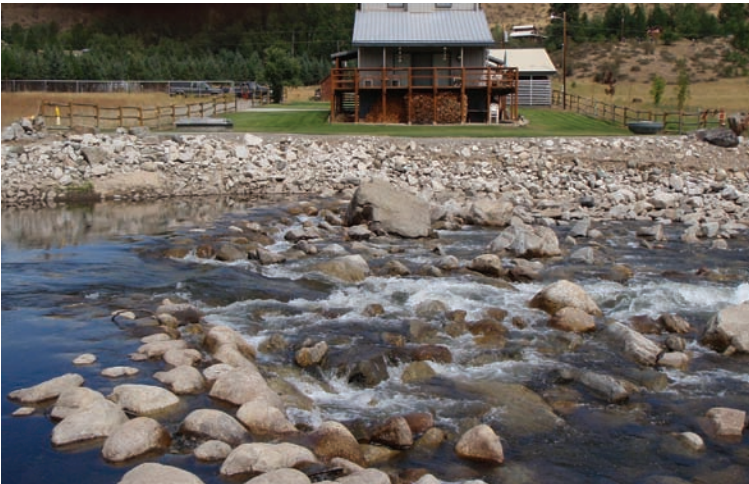
Crest of the new Fulton structure
