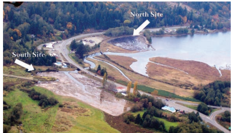
Overhead aerial of finished estuary construction sites at Salmon Estuary showing both the North and the South sites together. Note newly created tidal channels within both estuary areas
