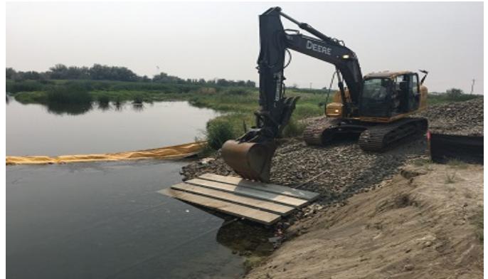
Access manager Josh Harmon constructing new boat launch at Winchester Wasteway.
