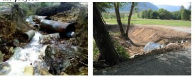
**Peterman Unit** — the complete failure of the 2500 road is still not repaired. The road is closed, sedimentation has been stabilized, and water is flowing through the culvert. The project has been accepted and funded as a FEMA project and is expected to be fixed in 2010. Other locations reported in the 2009 update were fixed and all of the 75 miles of road on the Peterman Ridge Unit will be brought up to Forest Practices requirements by 2015.
