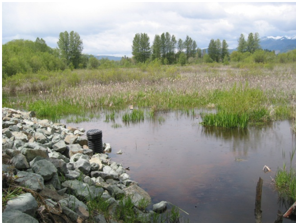
Standpipe to control water levels on Spears Unit
