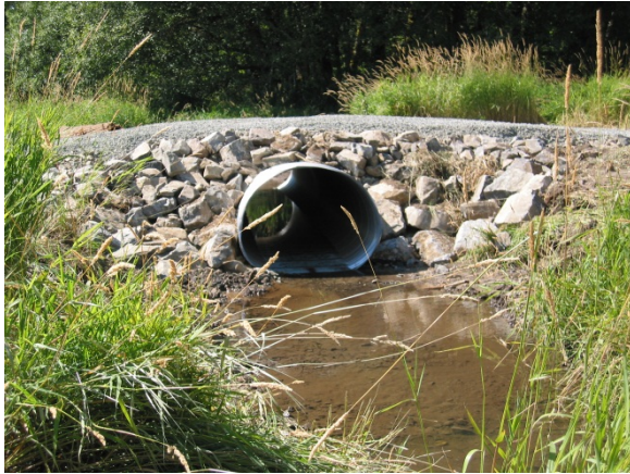
Culvert on the Kiona Unit replaced after flooding
