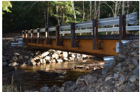
Bridge installed as RMAP culvert replacement
