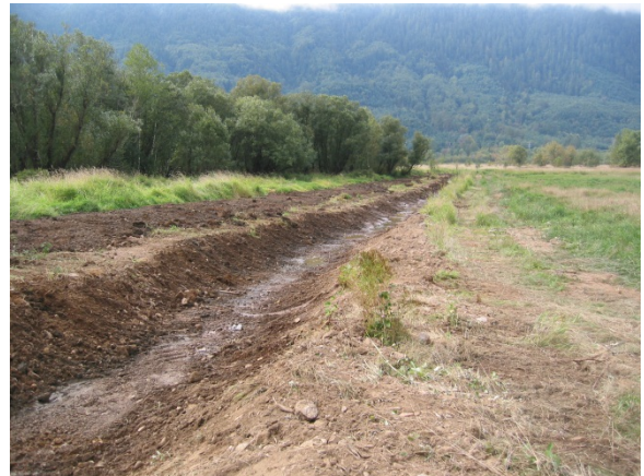
Davis Lake Field Drainage Maintenance Project
